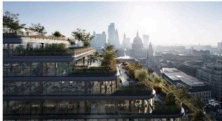
120 Fleet Street BIG England In Progress
