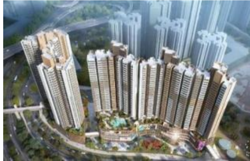
Kai Tak Area 1E1 site, Kai Tak (construction in progress)
